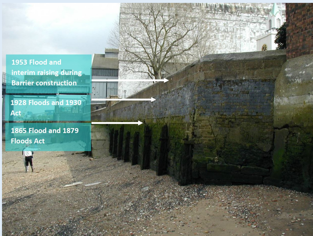
Figure 2: Historically a flood defence approach has led to “reactive” raising of the defences in response to major events – Courtesy Thames Estuary 2100 Project.
