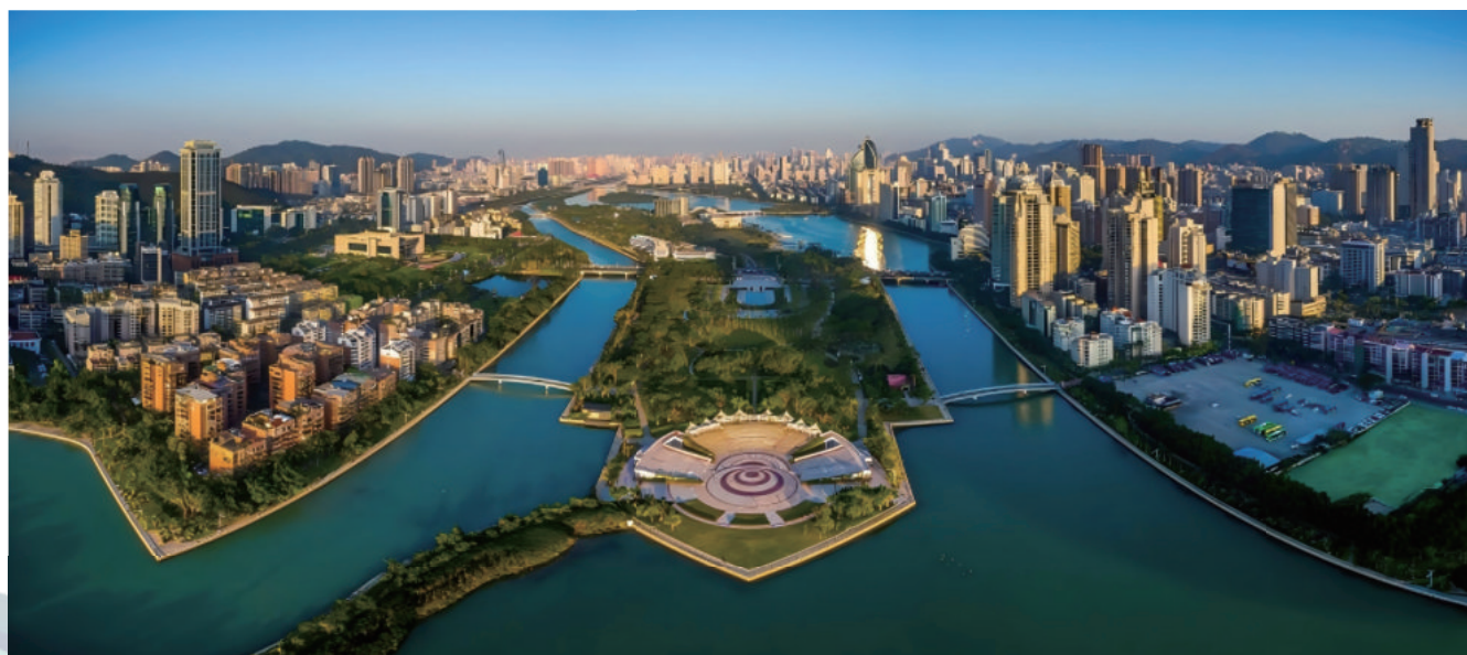
Figure 4-27: Aerial View of Yundang Lake
